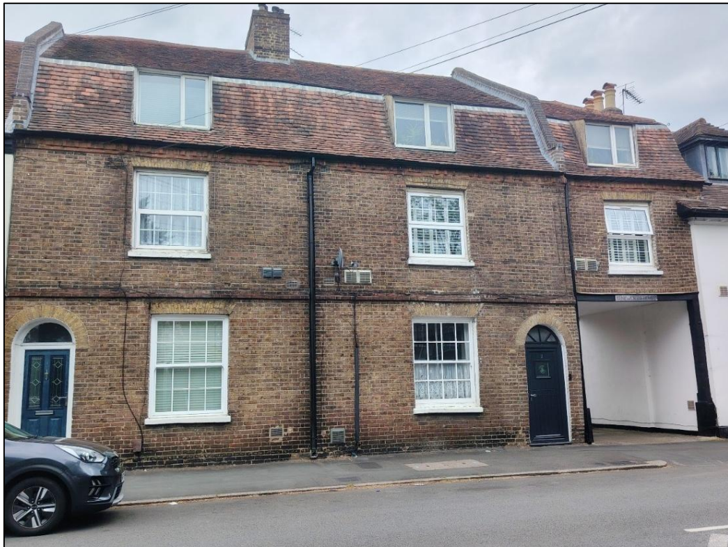
Kenilworth and adjoining house
