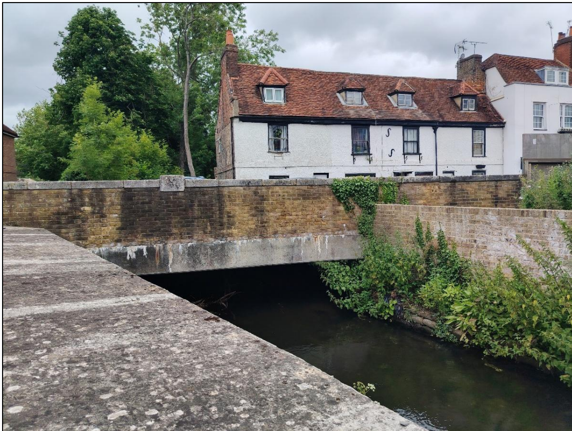
Colne Brook Bridge, 1,2 & 3 Park Street in background
