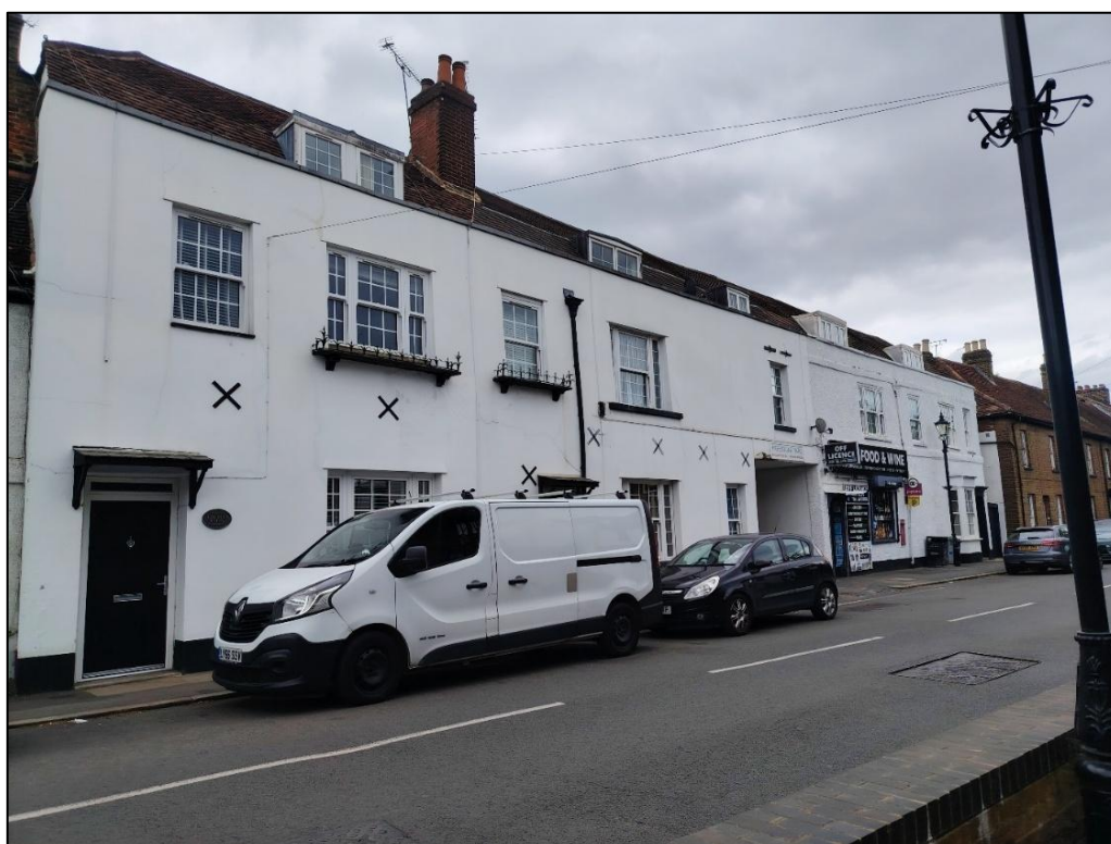
Badminton House, Post Office, adjoining house and Hampton House
