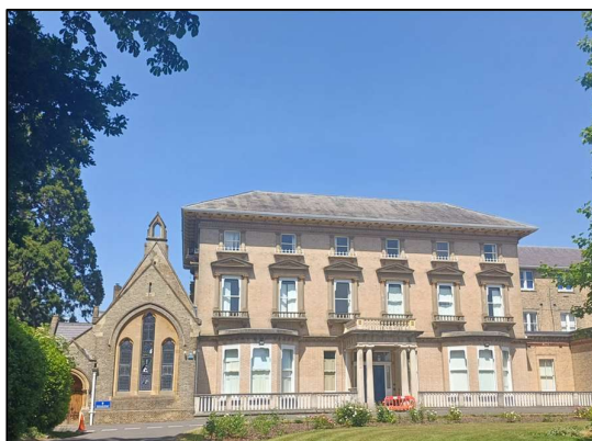
Front elevation of the grade II listed west block and Chapel at St Bernard's School
