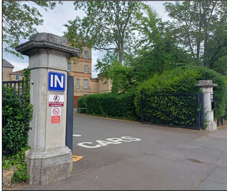
Stone gate piers at the entrance to St Bernard's School
