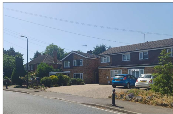
The property is not within the Conservation Area but the boundary runs across its front garden; the amount of hardstanding is not considered sympathetic
