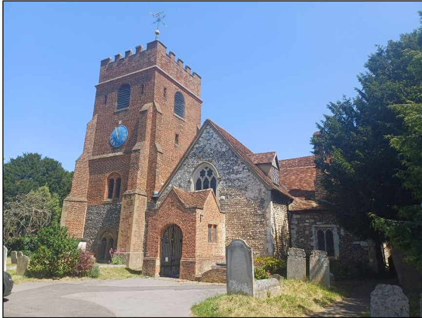
Red brick tower of St Mary's church
