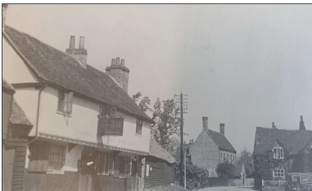
St Mary's Road, Langley looking north with the Red Lion on the left, the former Depree school beyond it. On the right side is the former Vicarage, both it and the school were demolished in the mid twentieth century as part of a road-widening scheme
