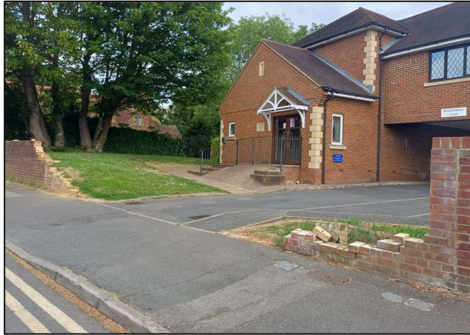
Damaged boundary wall to Mountbatten Court
