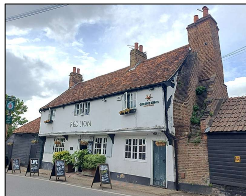
The Red Lion with timber frame visible in gable end
