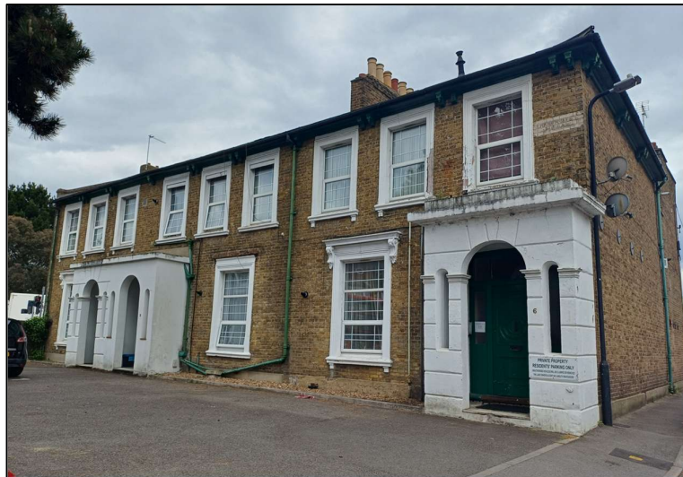
Numbers 6, 8 and 10 Clifton Road – yellow stock brick with stucco porches and window surrounds
