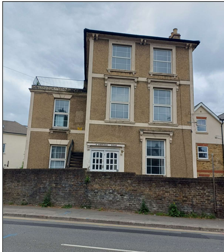
Nineteenth century boundary wall along Uxbridge Road
