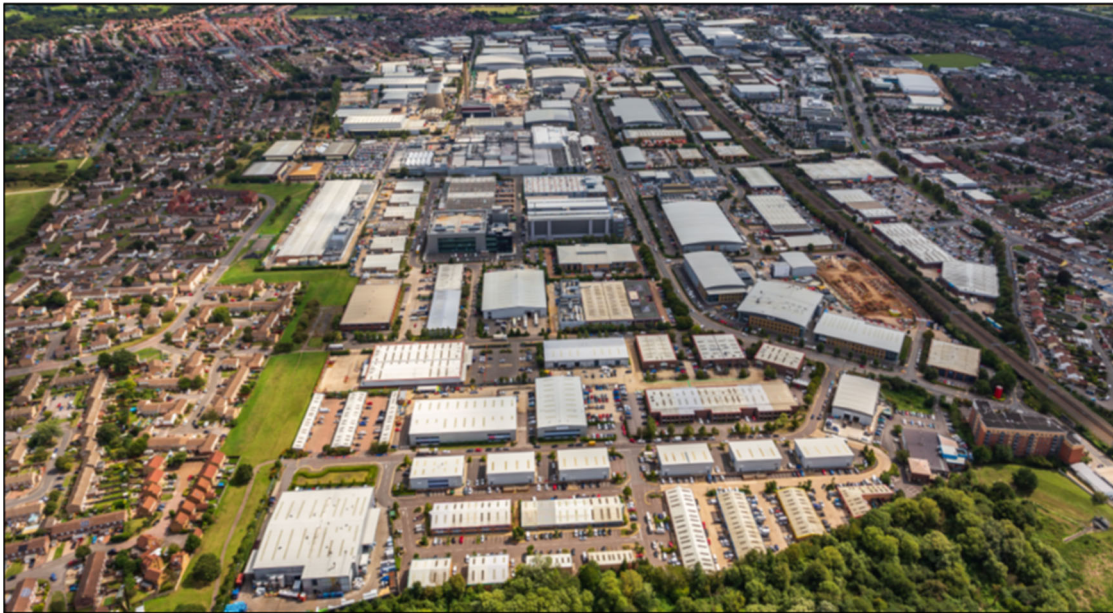
Figure 2.1: Slough Trading Estate looking east
