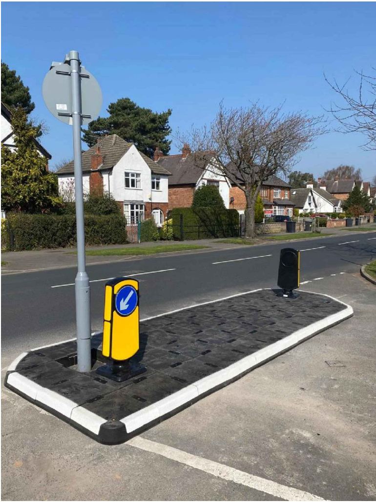
EXAMPLE OF ISLAND CONSTRUCTED USING REDIPAVE UNITS
